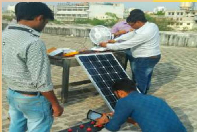
Practical Trg. on Installation and Maintenance of Solar Plant & Equipments
